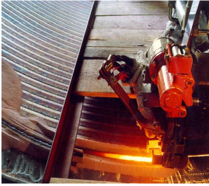
Figure 3: ESAC weld overlay in progress
