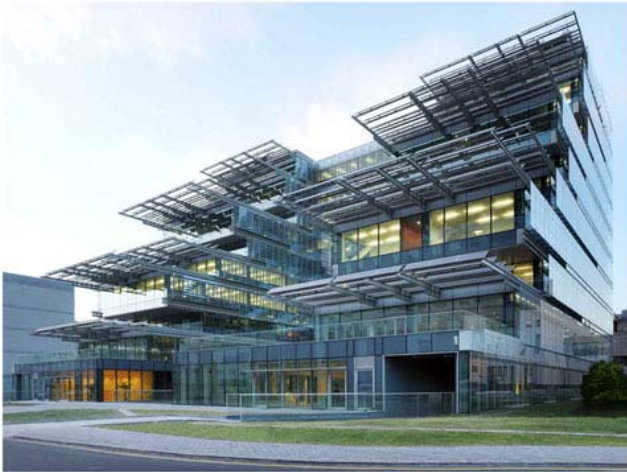
Fig. 6. SIEEB building, Beijing, China, 2006. PV modules are arranged as wings that perform as sun-shading devices and give form to a kind of semitransparent half-pyramid.
