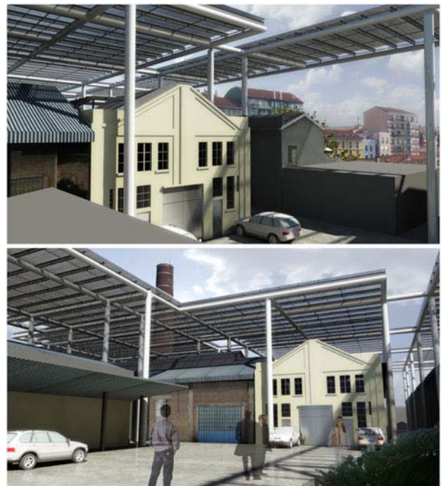
Fig. 8. The Roof project, Milan, Italy, 2010. PV modules are arranged in a semitransparent roof that covers a cluster of buildings.
